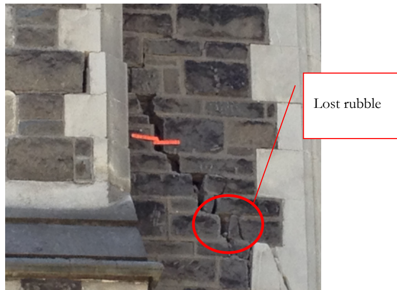
Figure 2: South transept wall, February 3, 2014
